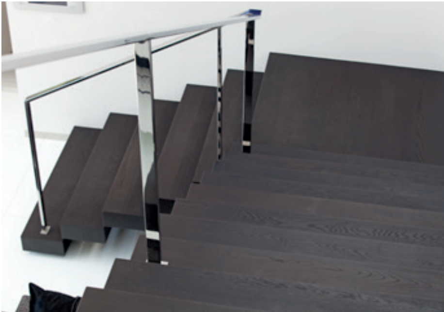
Cantilever staircase crafted from the same wood as the floor.
